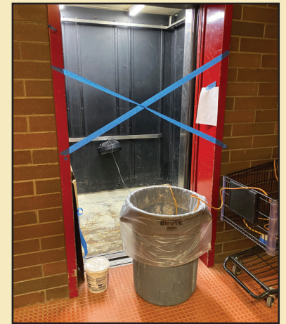
Elevator construction in the science building
